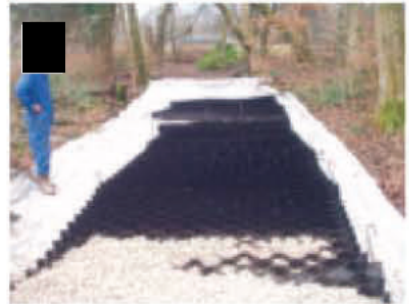
Installation of the CellWeb™ system.
